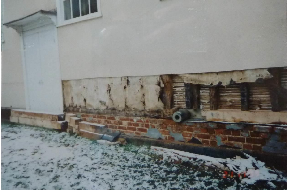
Figure 3: Repairs to the sole-piece in November 1993, showing the timber framing (Great Bardfield Meeting House archive)
