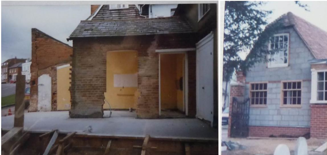
Figure 2: The demolition of the 1848 extension (left) in 1985 and the newly constructed extension before rendering (right) in 1986 (Great Bardfield Meeting House archive)
